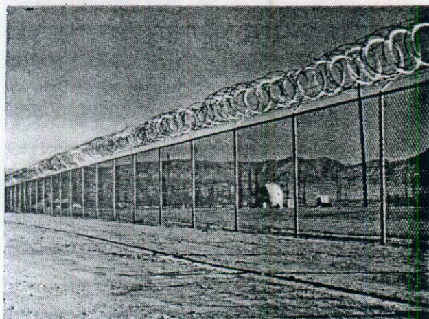
Figure 3-4. Alternate Security Fence with Single Roll 30/24 GPBTO. Upgrade Cost: $5/ft ($16/m) [FY 79].
